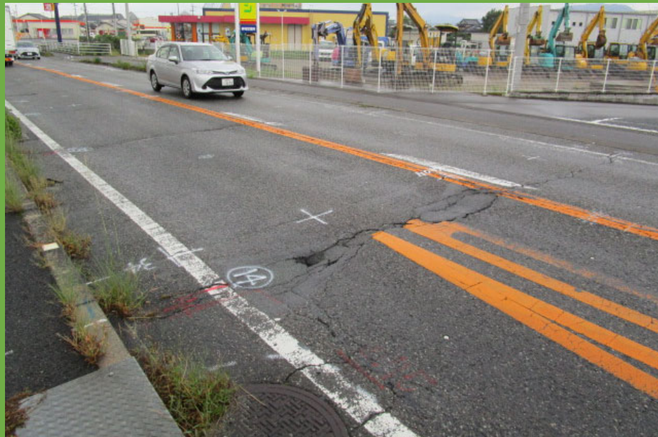
Before (通常の舗装)
