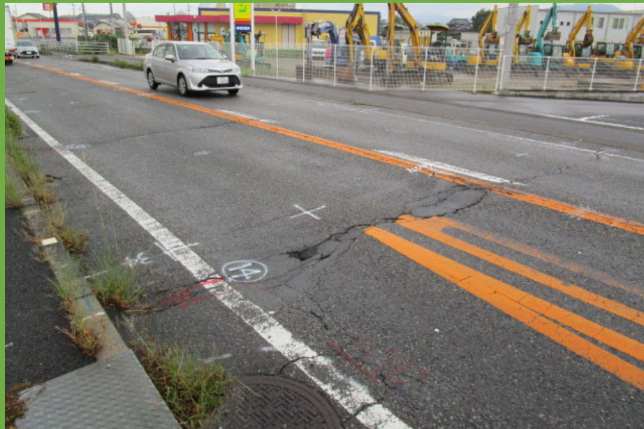
Before (通常の舗装)
